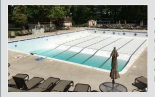
When the rain paused in early May, we were able to complete a major capital project by resurfacing (or white coating) the lower pool. Resurfacing is necessary investment and extends the life of the pool. At 10 years of age, it was the appropriate time for lower pool to be resurfaced.
